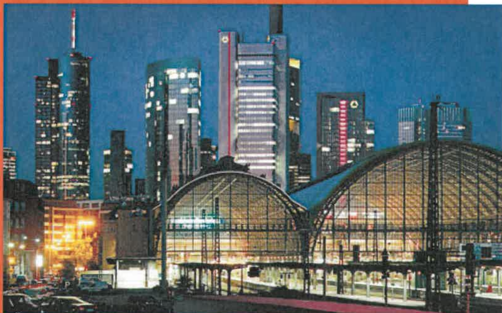
Railway station in Frankfurt am Main
